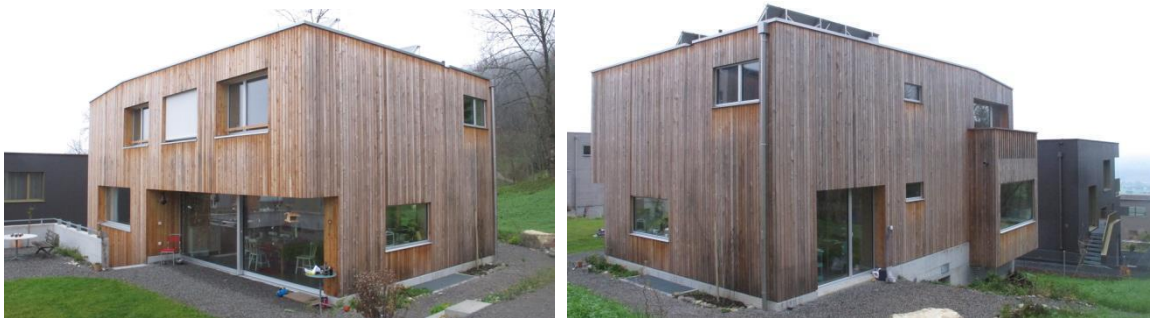
Figure 1: Measurement object is a Minergie-certified standard wood construction in Rickenbach, Switzerland (left hand, south-oriented face; right hand, north-oriented face )
